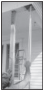
1. Measure opening where post will be installed.
