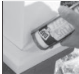
12. Slide skirt into position and caulk seam.
