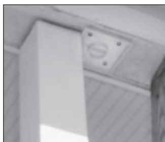
5. Position top of post directly under the top fastening plate.
